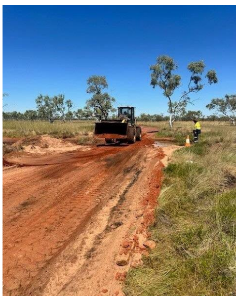
Figure 1: Kundat Djaru (Ringer Soak) Floodway Crossing repairs
