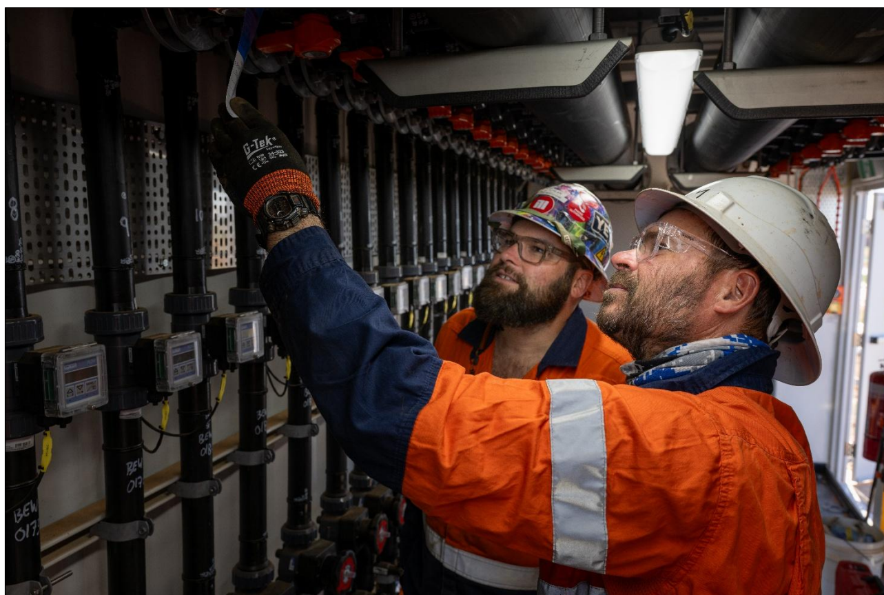
Figure 25: Photo of Boss team working inside the wellhouse
