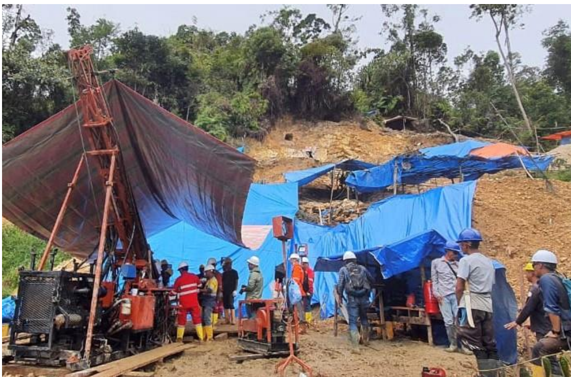
Figure 3: Image showing drilling commencing at Anak Perak prospect on 18 September 2022.
