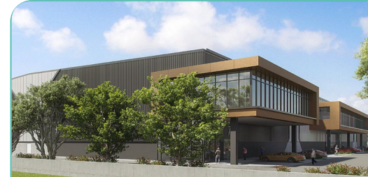
12 Church Road, Moorebank NSW 2
