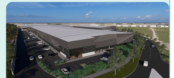
19 & 21 Pilatus Street, ASCEND at Jandakot WA 2
