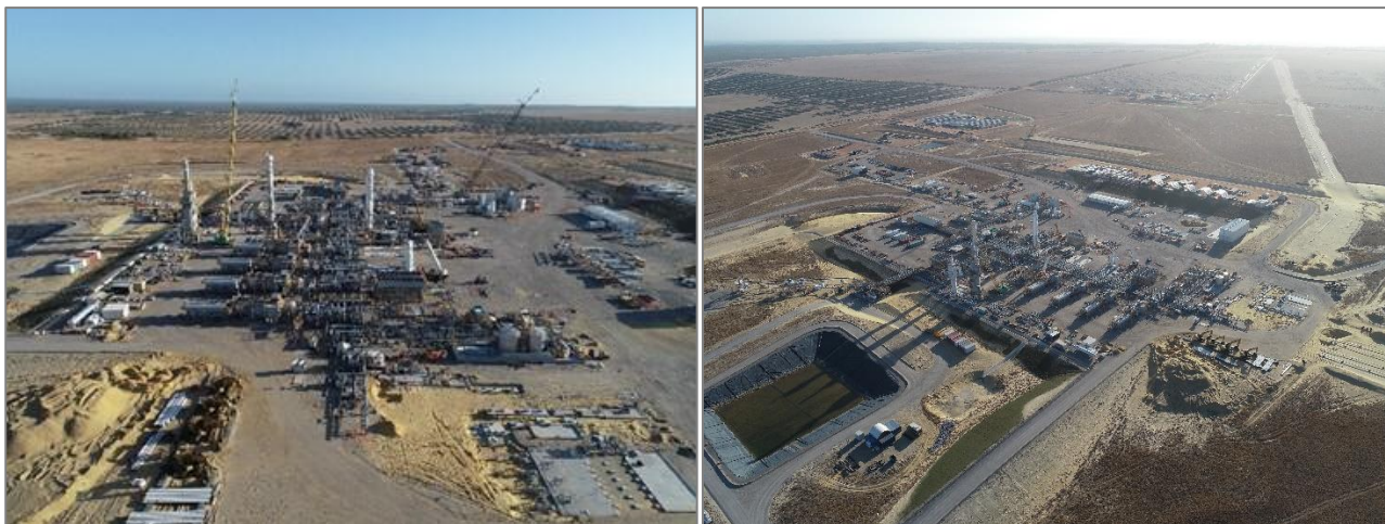
Waitsia Gas Plant construction (February 2023)
